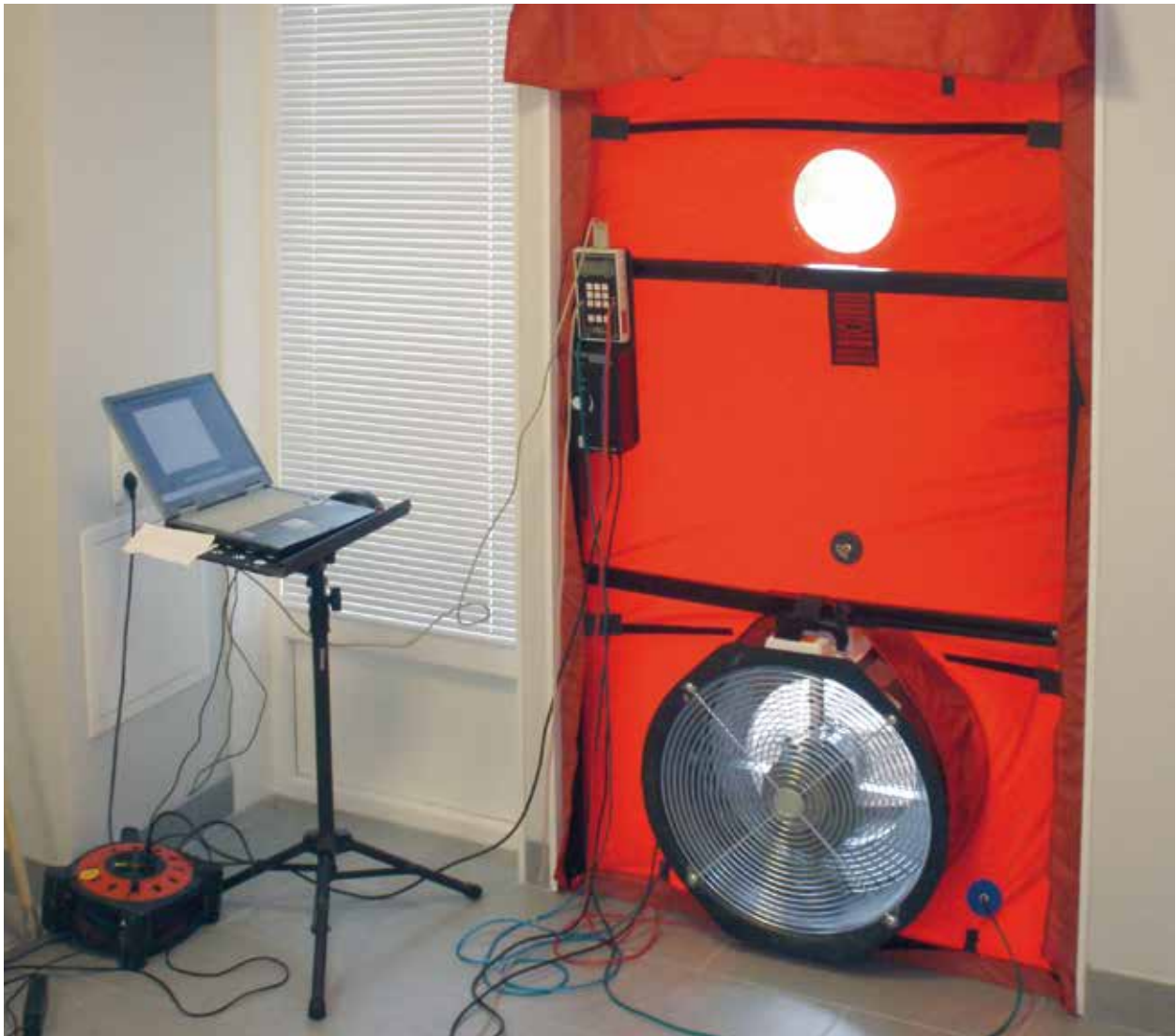
Airtightness measurement detects the building leakage points even before the sealing of structures
