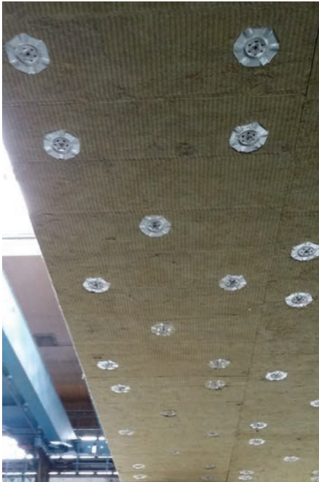
Fire protected concrete slab.
