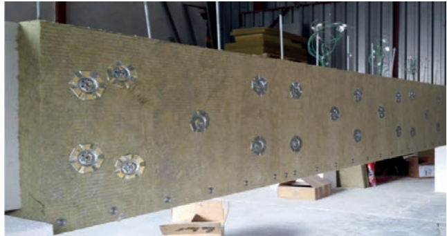
Fire protected concrete beam.
